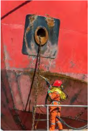
Hull Sandblasting
